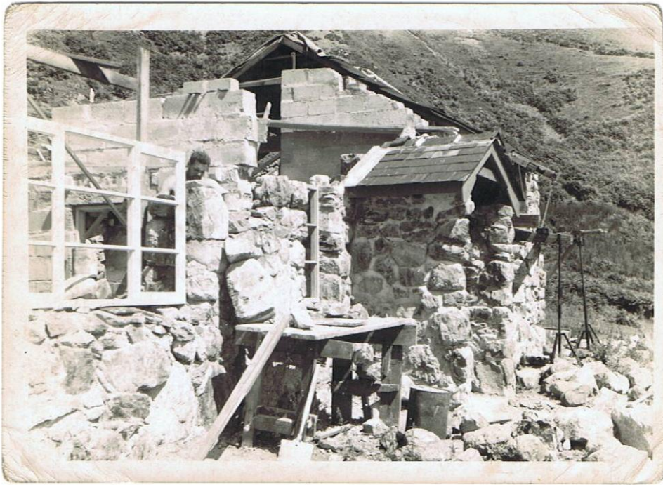
Building the Sitting Room Wall (Bryn Hafod) – submitted by Nick Smyth
